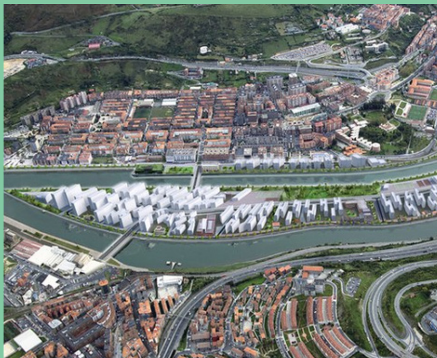
Above: Aerial picture of Zorrotzaurre peninsula. Below: Impression of Zorrotzaurre island after the redevelopment. ©Comisión Gestora de Zorrotzaurre
