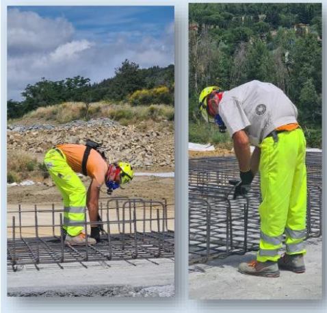
Tying of reinforcement bars
