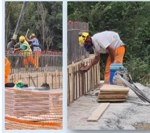
Vibration of the concrete jet and cleaning of the concrete removed from the formwork.
