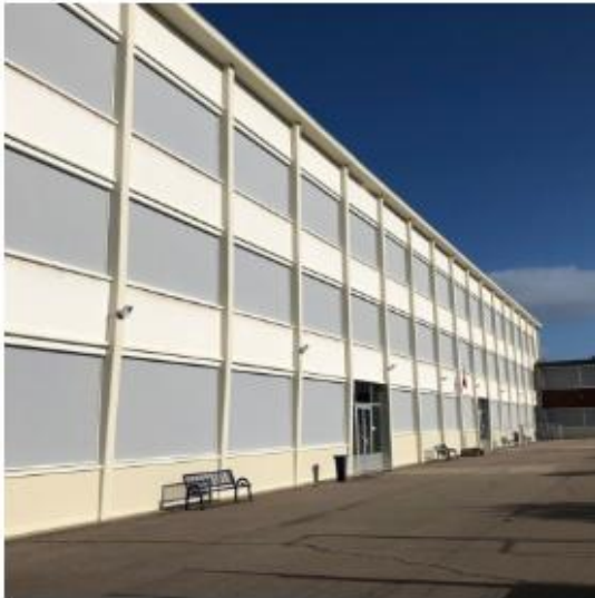
Install sun protection (shutters, blinds, ...)
